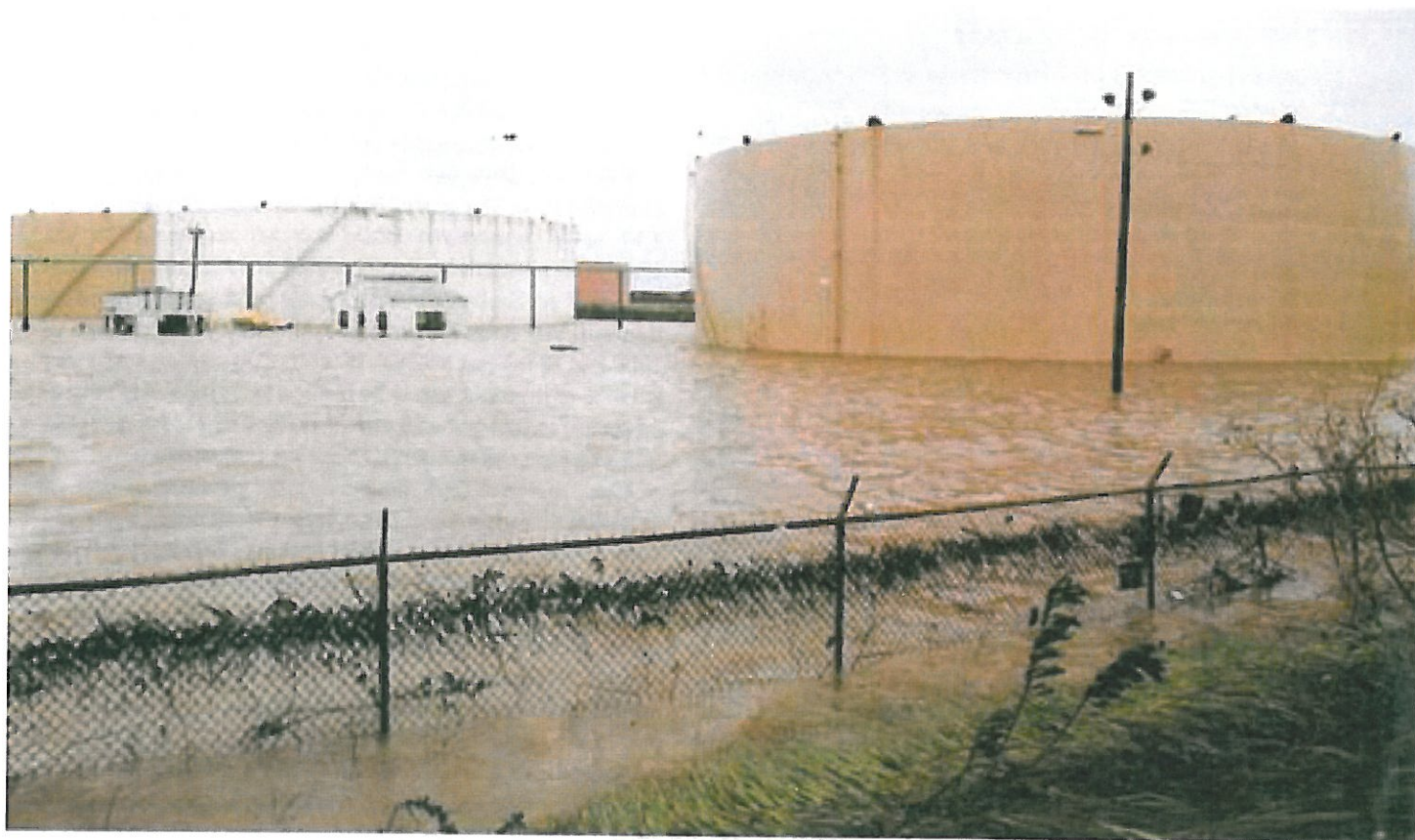
Storm waters flooded these petroleum storage tanks near Mobile, Ala.
